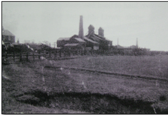
3.8: Marston Pool mine seen from the south, showing a new subsidence hole beginning to form 21
