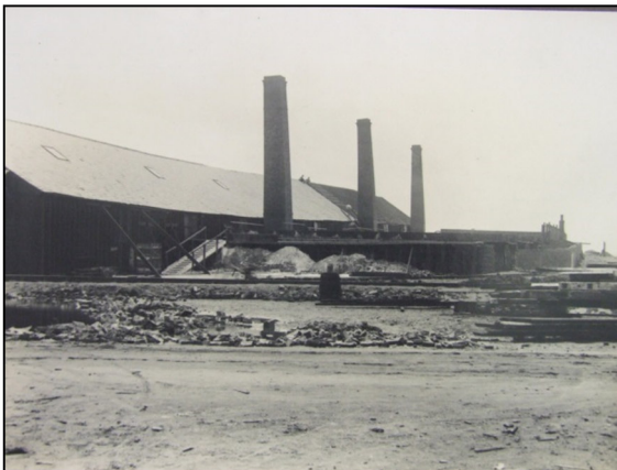
3.15: The Adelaide Works in 1928. A bank of common pans (on the right), with attached store houses (on the left) and rows of chimneys. This was typical of larger works. 49
