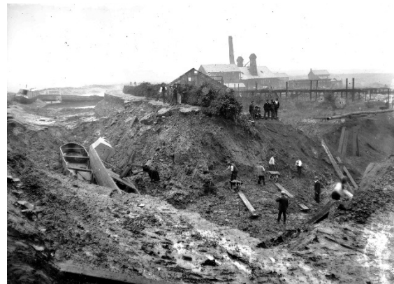
3.7: Marston Hall Mine, after the collapse of the mine and breach of the canal in 1907. The picture faces north and the turn of the canal can be seen in the background. The buildings beyond the breach are the mine buildings in the north-east of the site
