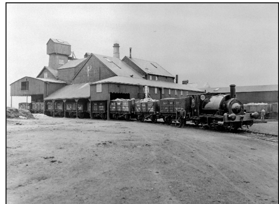
3.13: A Salt Union locomotive shunting wagons by the pit head gear of the Adelaide mine. There is a canal arm immediately behind the locomotive. The covered 'sheds' over the pit head gear were to prevent rain water entering the mine and dissolving the rock salt. 46
