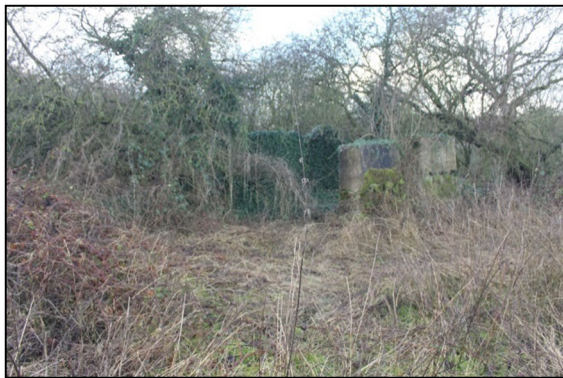
3.16: The pit head of the shaft to the rock salt mine is marked by a series of concrete blocks and protected by steel railings, these are located south-west of the Adelaide Flash
