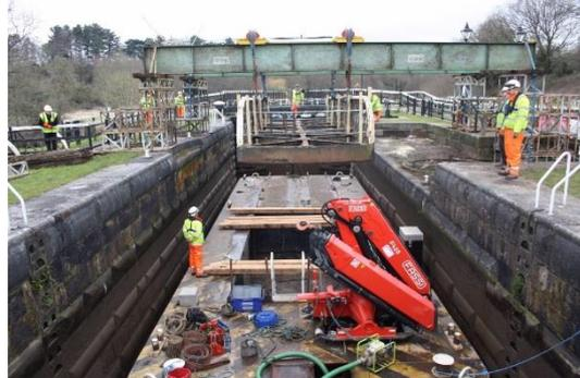
The renovation work involves cleaning, shot-blasting and priming to prevent further corrosion, before the bridge is put into storage for 12 months. The second phase of the renovation works, depending on available funds, would be in spring 2017 and include extensive repairs and re-painting of the structure.
